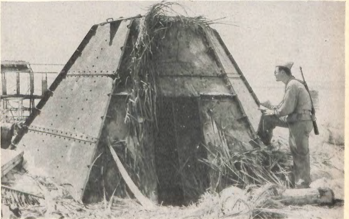
Figure 145. A hexagonal steel pillbox.
